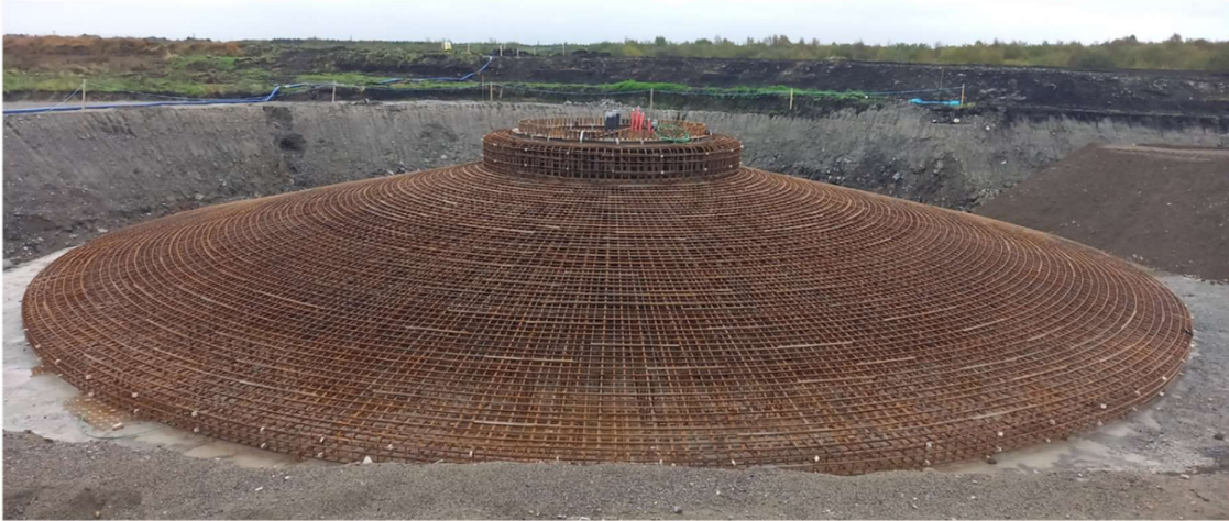
Plate 3.3: Completed Turbine Base Cage
