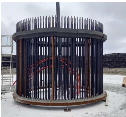
Plate 3.1: Levelled Turbine Anchor Cage
