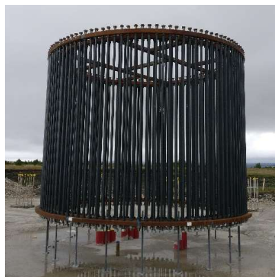
Plate 3.2: Turbine Anchor Cage with Adjustment Feet
